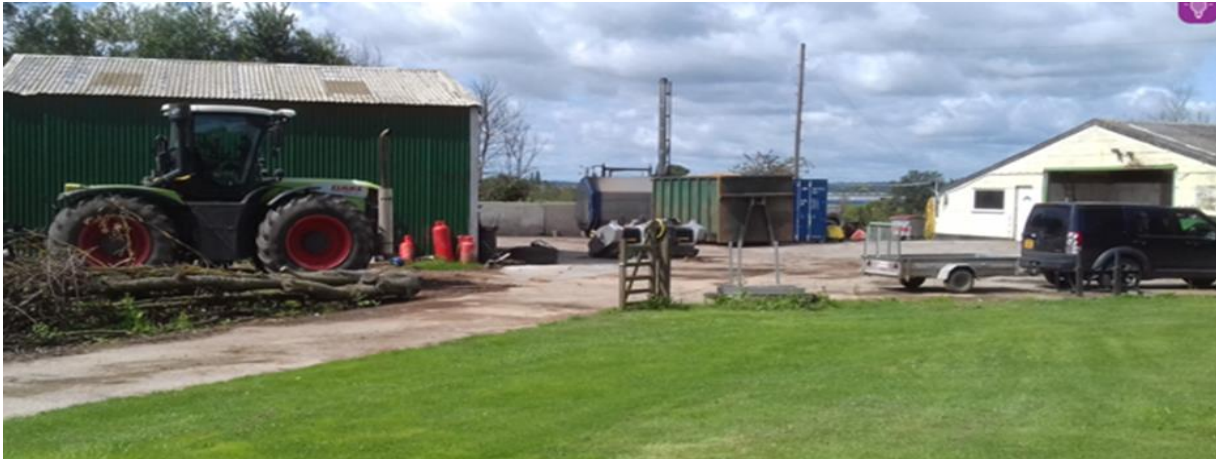
Photo taken on site of the boiler (and control room) and drying containers with two existing agricultural buildings either side – with 4m high flue (summer of 2022)
